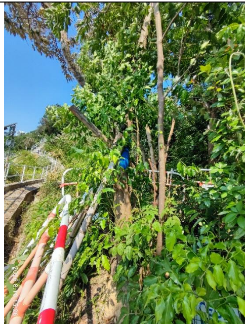
T8231– General view
